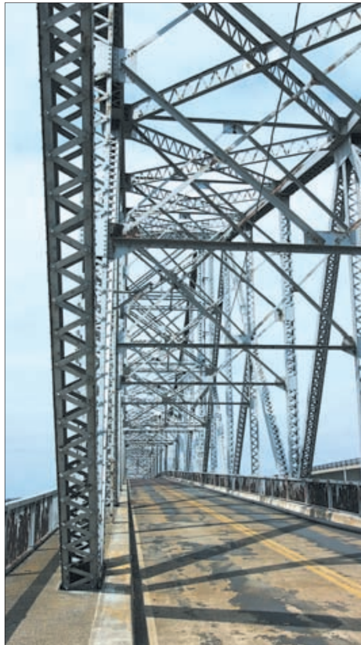
Work is expected to begin next week on the demolition of the old Jamestown Bridge, more than a decade after its use was suspended because a new bridge was built.
