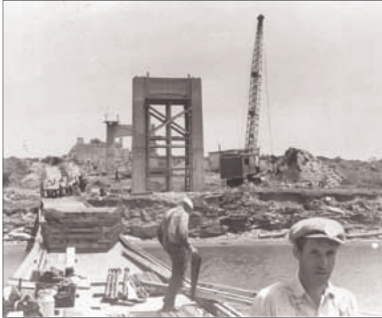
Construction of the old Jamestown Bridge.
