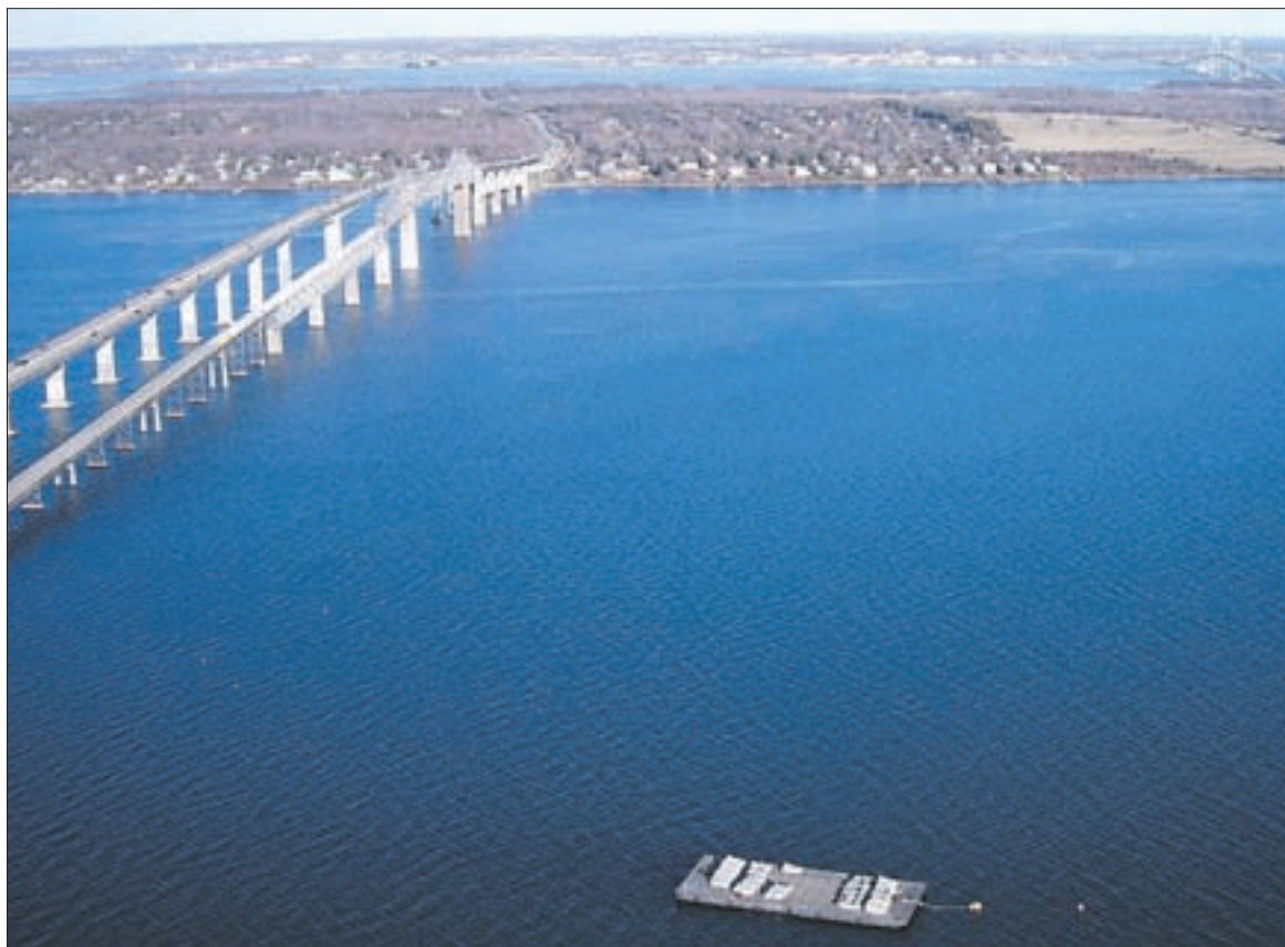
State DOT officials say it will take three explosive "events" to demolish the old Jamestown Bridge. This aerial photo was taken Monday evening by Nate Bousquet.
