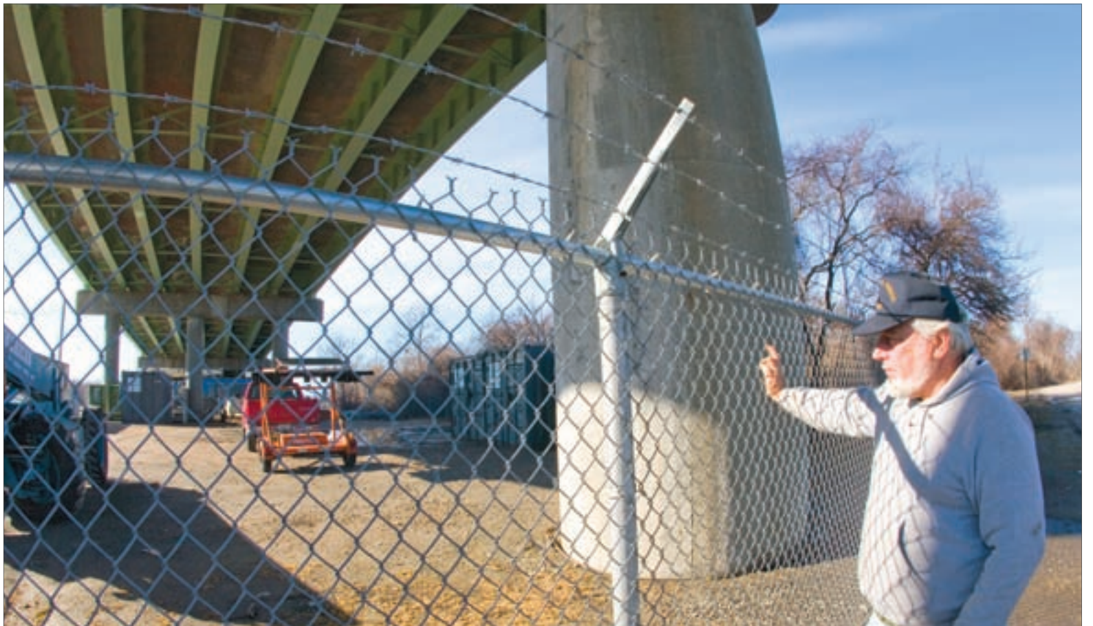
Nick Robertson looks at the Pell Newport Bridge maintenance site on Freebody Lane where he believes paint solvents were buried during the 1970s. Rhode Island Turnpike & Bridge Authority officials say they are investigating Robertson's allegations but have found no evidence of chemical dumping.
