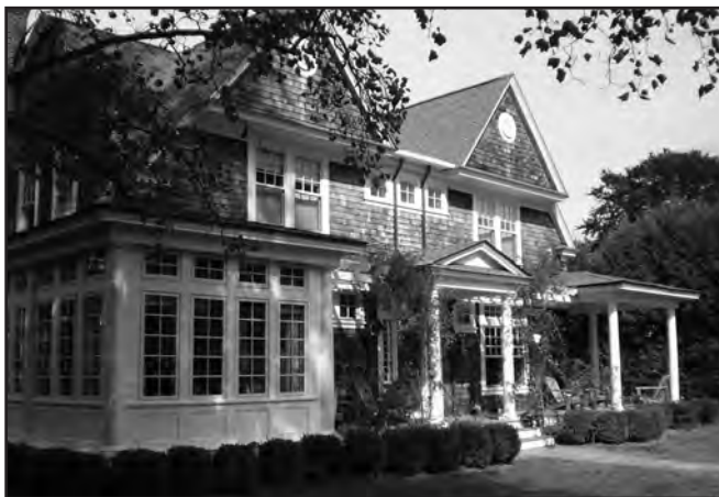
100 Longfellow Road Shoreby Hill, Jamestown
