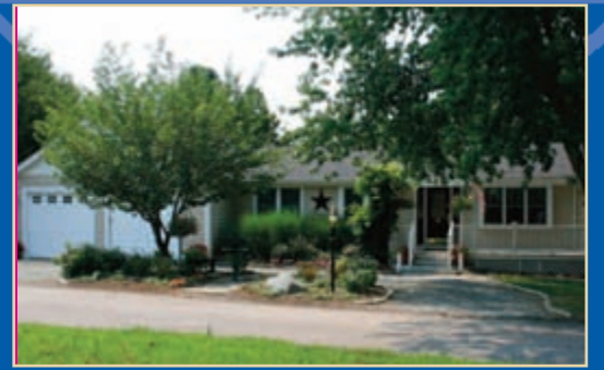
Jamestown-Open Sun 1-3PM 7 Port Ave. "Classic renovation" 3 beds, 2 baths, lower level guest quarters/in-law apartment. More house than meets the eye. $774,900 423-3440
