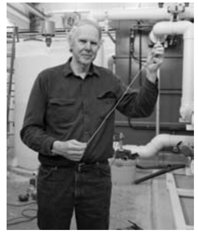
Steve Goslee holds a sample filtration tube that is used to clean Jamestown water at the new plant. Thousands of these tubes are needed.
