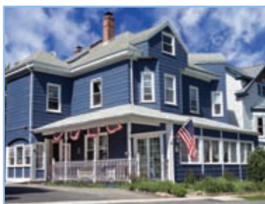
VICTORIAN VILLAGE HOME NEAR THE HARBOR $895,000
